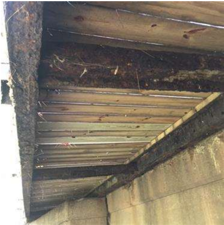
Sidewalk girders with pitting and laminar rust
