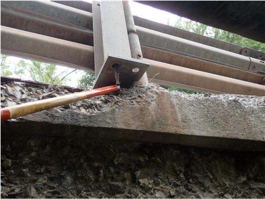
South railbase spall undermining H post
