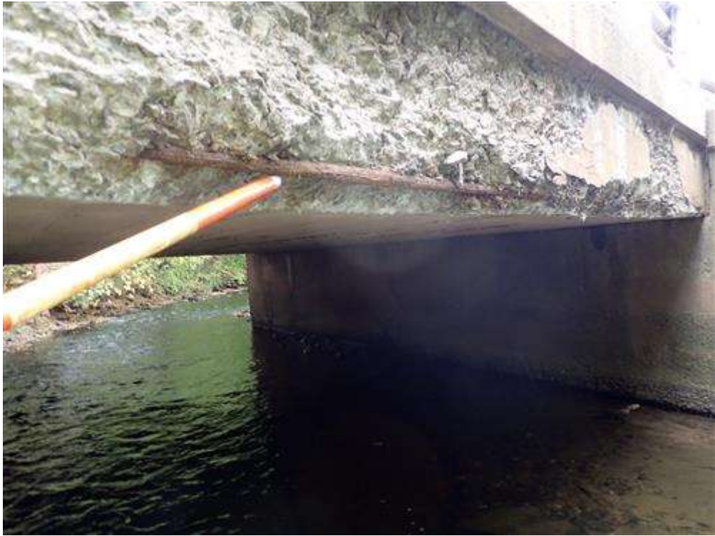
South railbase severe scale with exposed rebar
