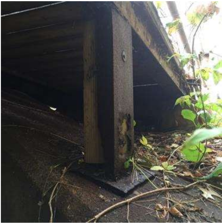
Steel H posts sidewalk supports with perfs at northwest
