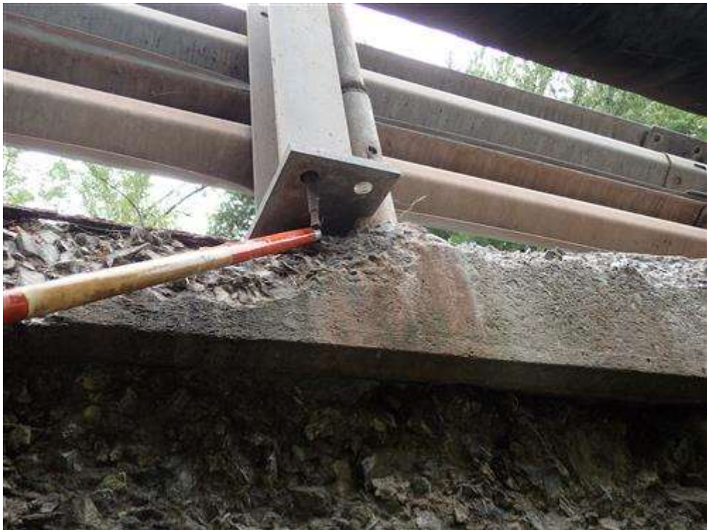
South railbase spall undermining H post
