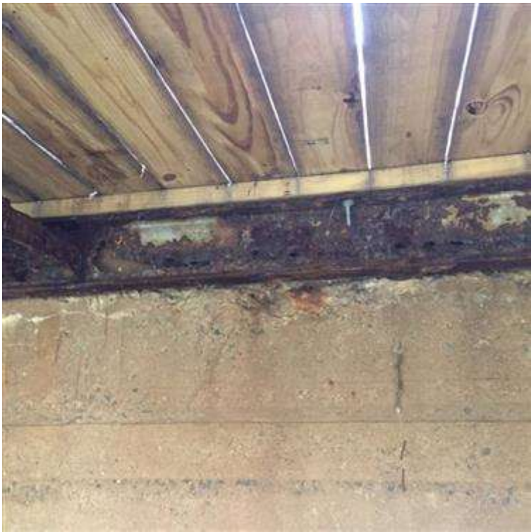
Sidewalk cross diaphragms with several perforations in web area
