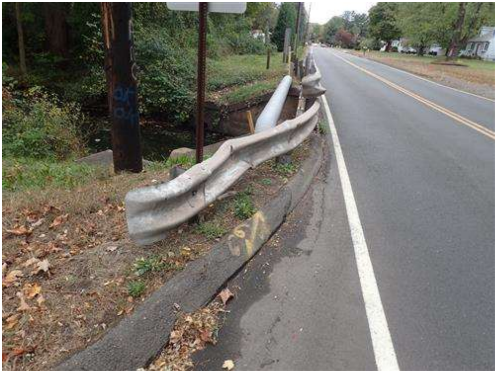
Collision damage at southeast M.B,R
